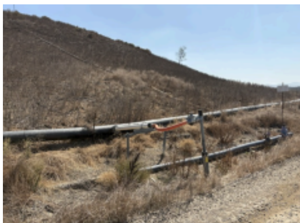
Photo 1: Landfill Gas Well (taken by A.Causey)
