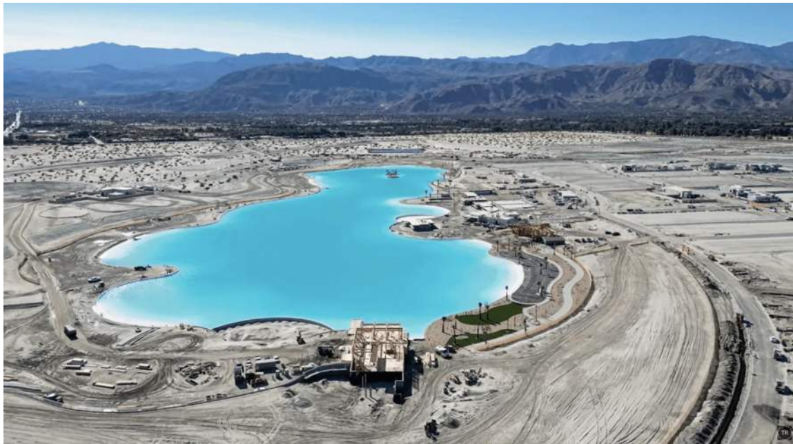
Figure 2: Cotino lagoon during construction, December 2, 2025 Source: Crystal Lagoons
