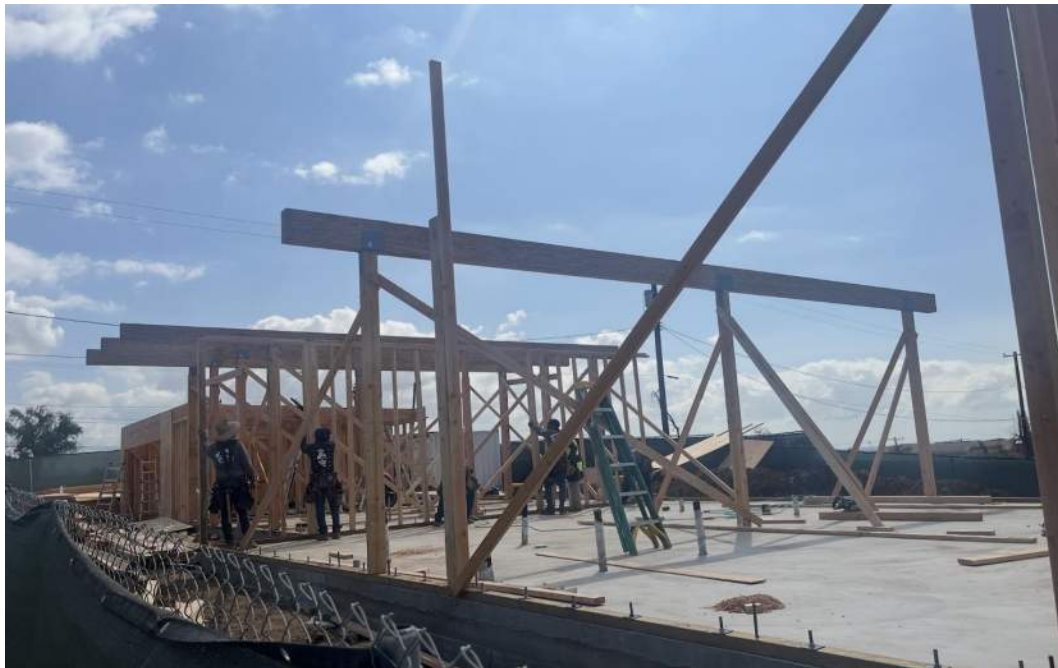
Reconstruction of my new home is in progress.
