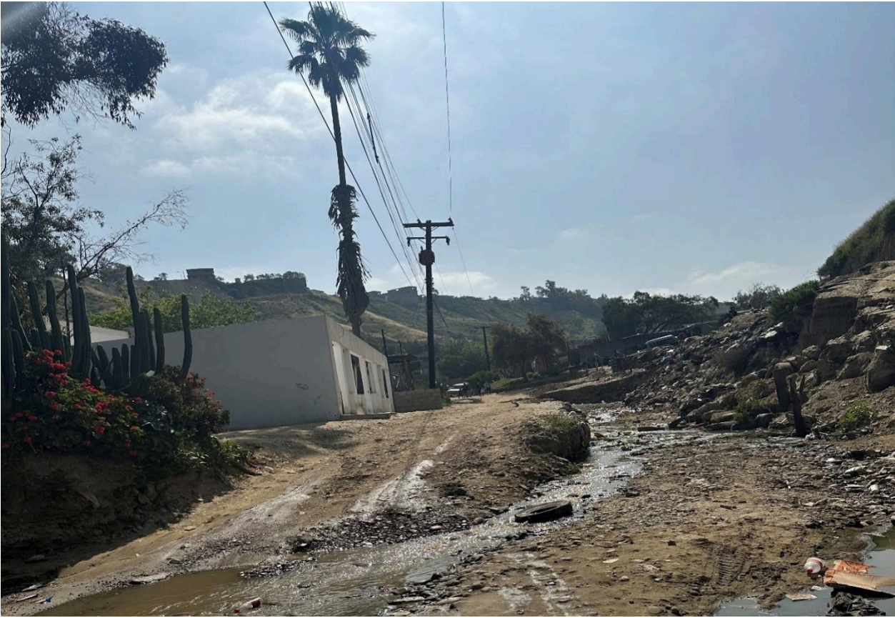
Image Nine: A washed out road along South Fork Tijuana River.
