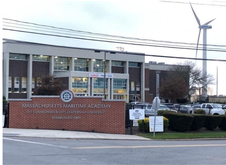
Wind Turbine Along Coast of Massachusetts Maritime Academy Property. Source: V. Taylor, 2024
