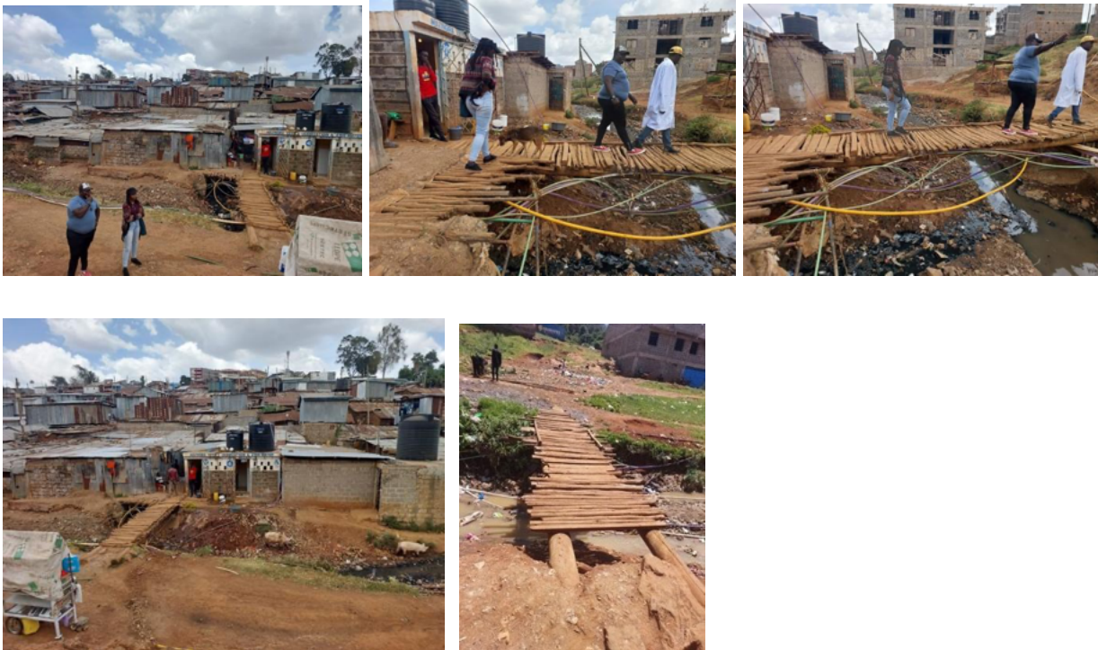
Figure 10 Various bridges constructed over the river by community members by repurposing electric poles
