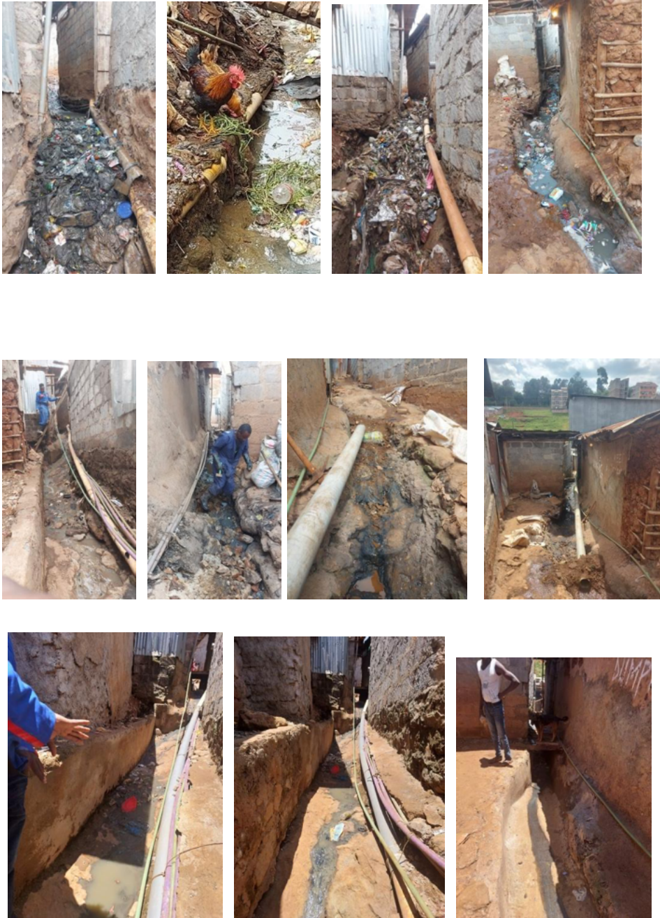
Figure 7 Before, during-construction, and after-construction images of a resident-led drainage initiative
